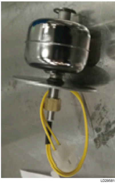
Figure 43: Density meter for low-chilled water supply type chiller
