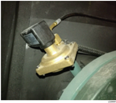
Figure 41: Level switch
