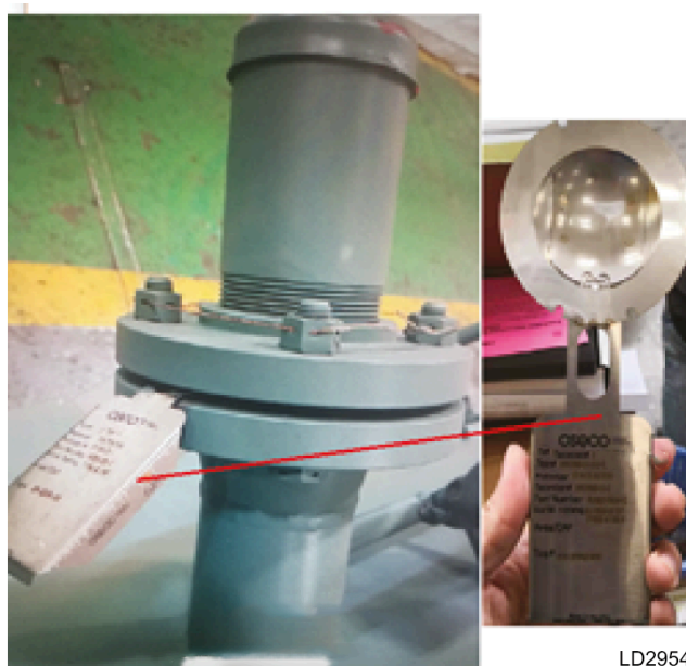
Figure 23: Oseco rupture disc kit
