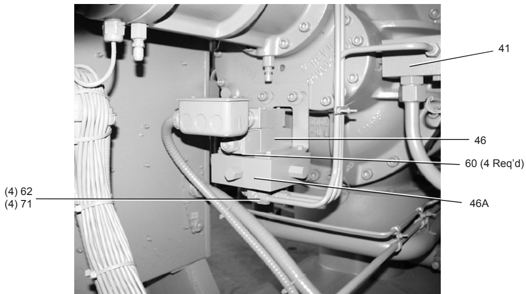
FIG. 8 – 4-WAY SOLENOID VALVE AND SUBPLATE
