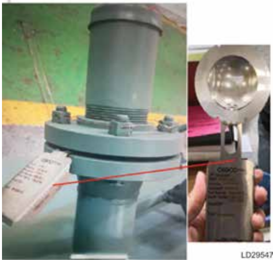
FIGURE 22 - RUPTURE DISC KIT AND RUPTURE DISC
