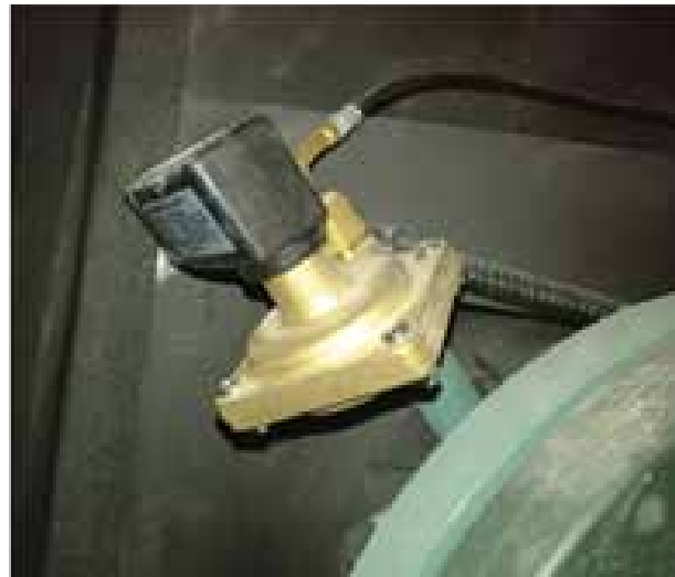
FIGURE 34 - PRESSURE DIFFERENTIAL SWITCH
