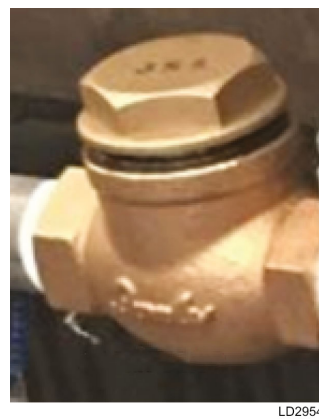
Figure 23: Check valve
