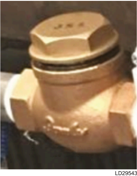
Figure 23: Check valve
