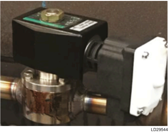
Figure 25: Sampling valve
