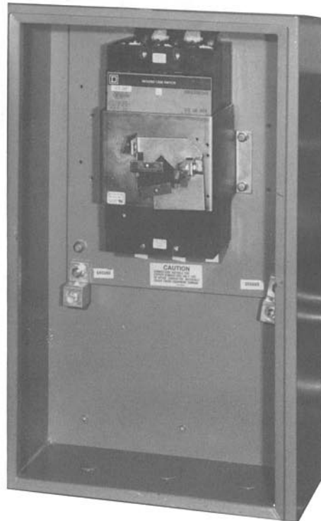
FIG. 2 – POWER DISCONNECT SWITCH (OPTION)
